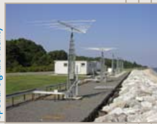
Transmitter antennas at the Special Signals Facility
